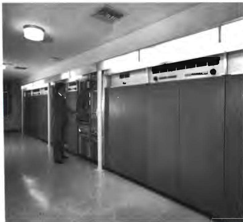
Chief Engineer Bill Yordy checks operation of KCST's twin 55 kW transmitters
